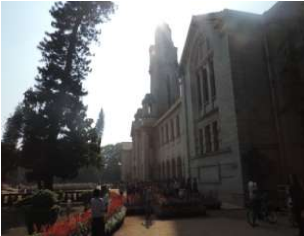
The Administrative Building, Indian Institute of Science
